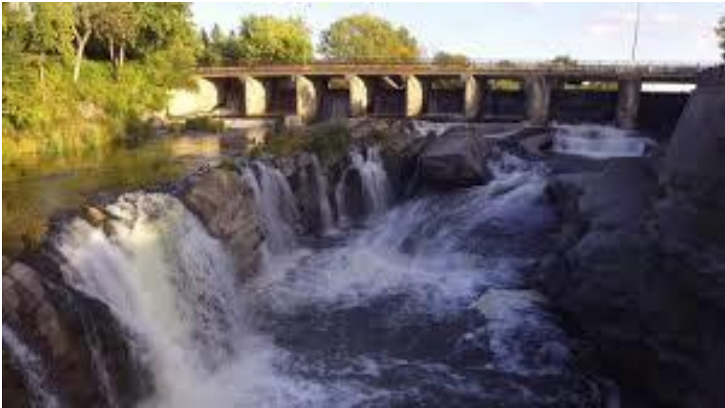
Hog's Back Bridge – Opened 1977
