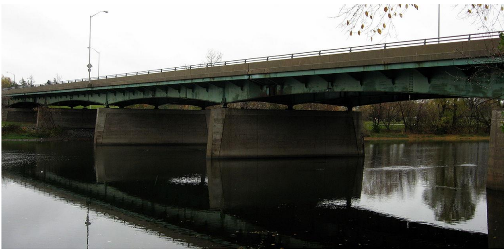
George McIlraith Bridge (Smyth Road) opened in 1966
