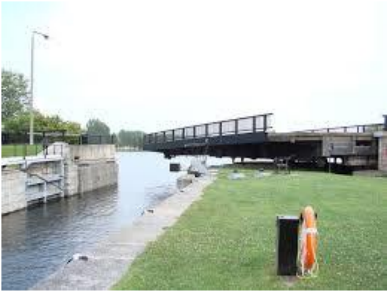
Hog's Back Swing Bridge
