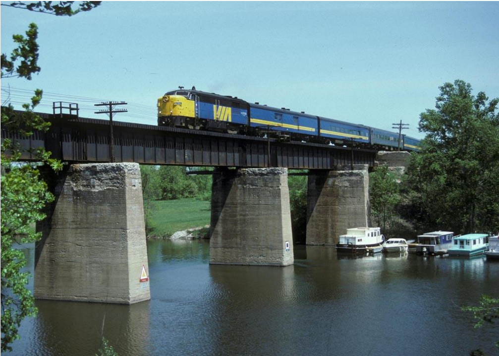
Canadian Northern Railway Bridge – Opened 1914
