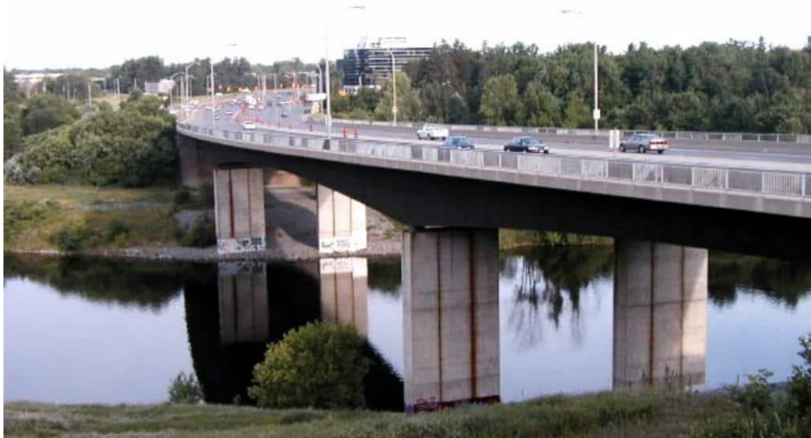
Hunt Club Road Bridge (Michael J.E. Sheflin Bridge) – Opened 1985
