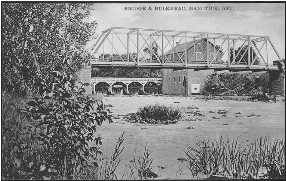
Manotick West Channel Bridge 1889 – 1958
