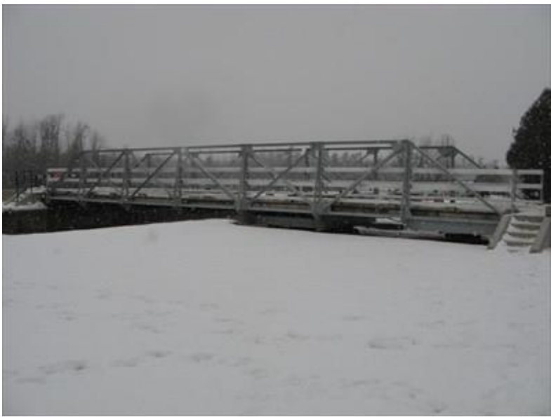
Nicolls Island Bridge and Long Island Locks
