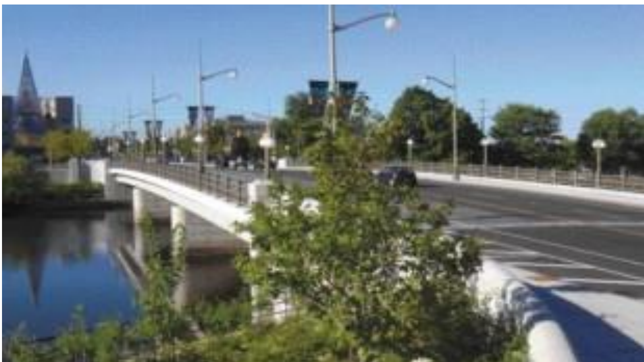
Bytown Bridges – Opened 1954
