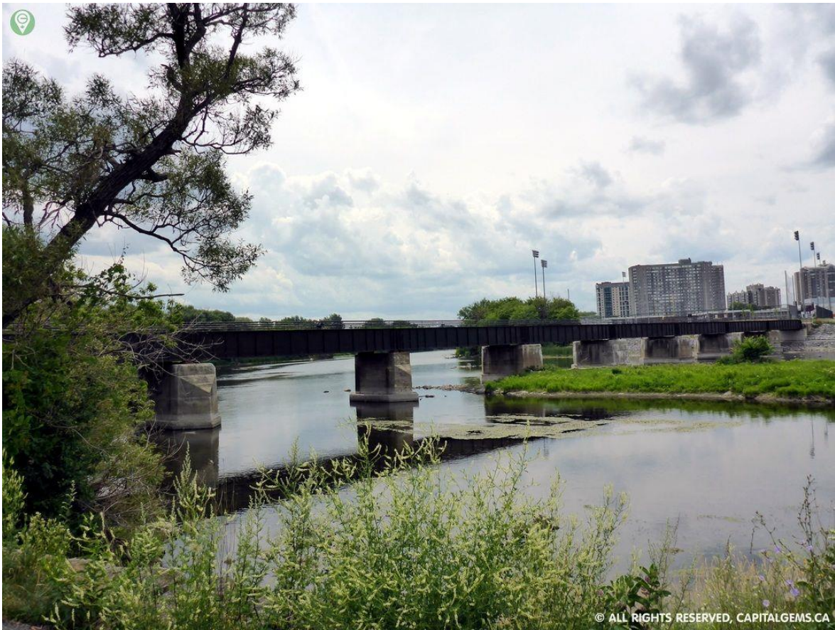
Former CPR Hurdman Bridge
