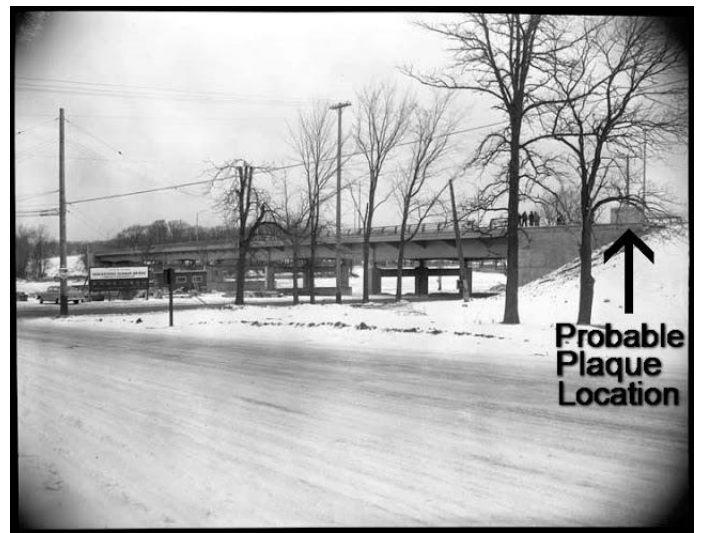
Dunbar Bridge opened 1955
