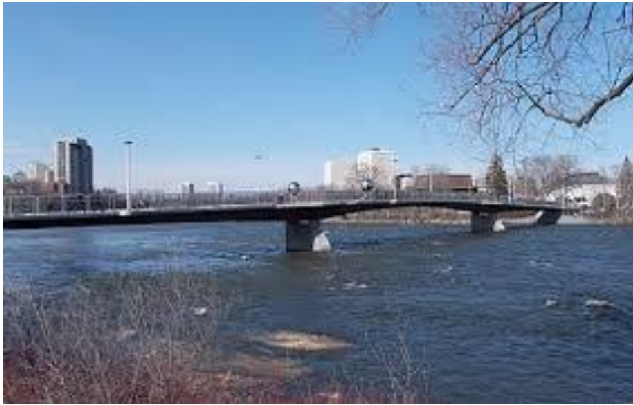
Adawe Bridge opened 2015
