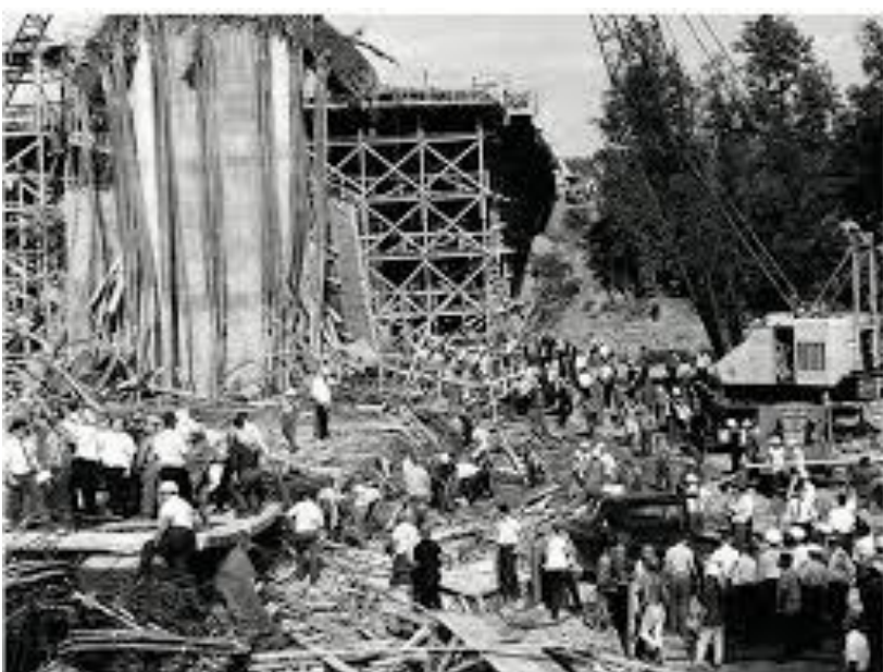
Heron Road Bridge collapse – 1966
